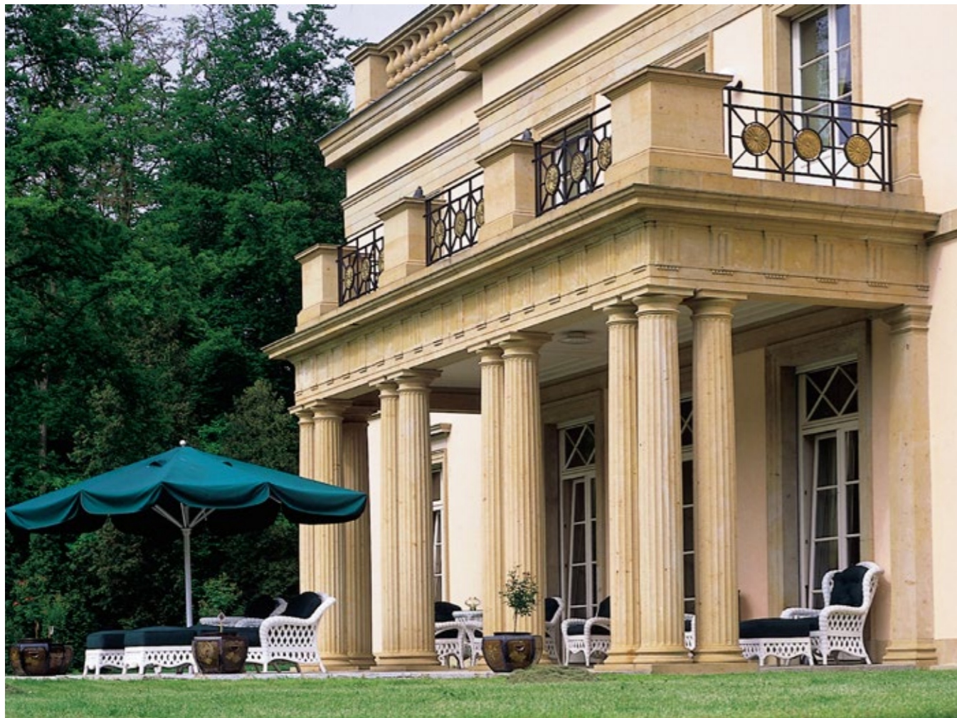
REINHARDTSDORFER SANDSTEIN, private Villa, Frankfurt am Main
